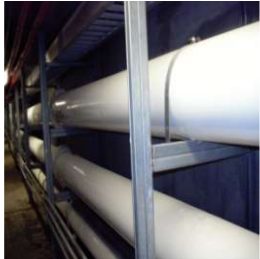
(Before and After: Section of Phase 1 work.)
