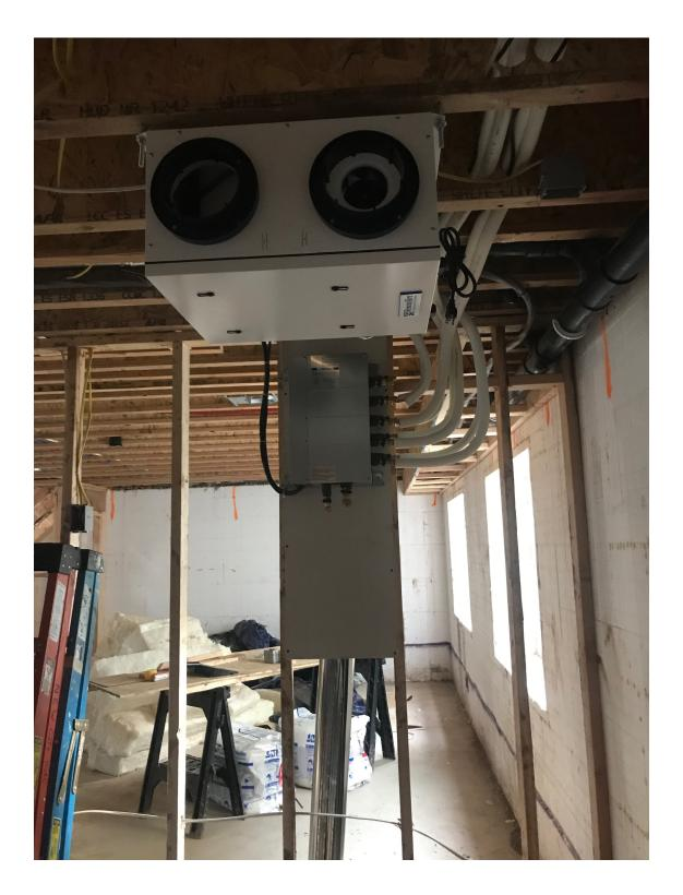
Traditional bathroom exhaust fans are replaced with exhaust air registers that are pulling 50 CFM of air out of the bathrooms/laundry constantly. The energy in this conditioned air is bypassed through a coil that transfers that energy into fresh air being pulled through the ERV and distributed into the common areas of the home.
