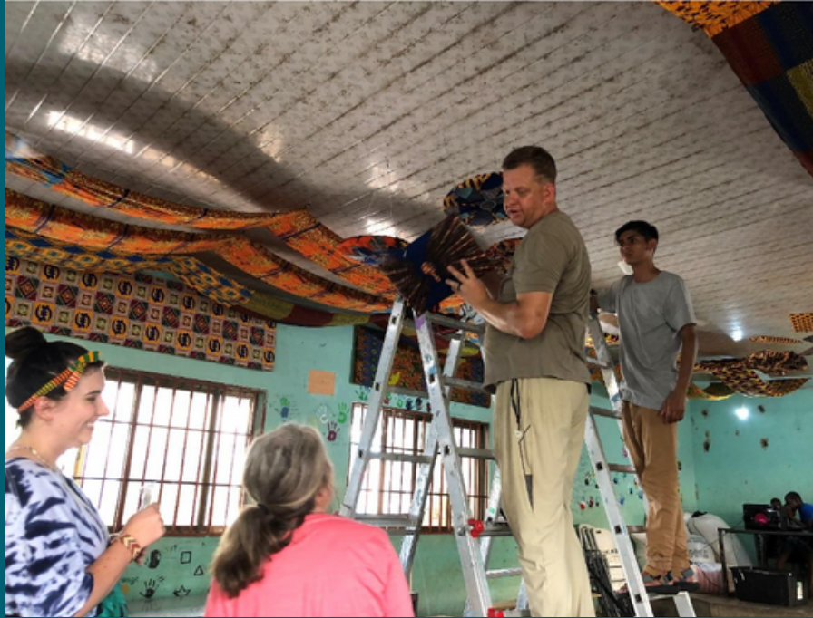
Installation of African fabrics and panels for noise reduction in buildings
