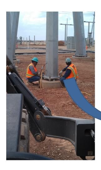
Fernando and Crespin attaching the nuts to the anchor bolts, securing the steel to the pier.
