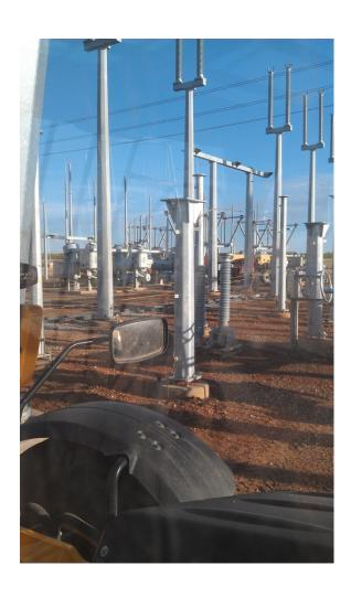
CCVT steel: 54 on site worth 2 hours. 13 feet 11 inches tall without the two part insulator.
