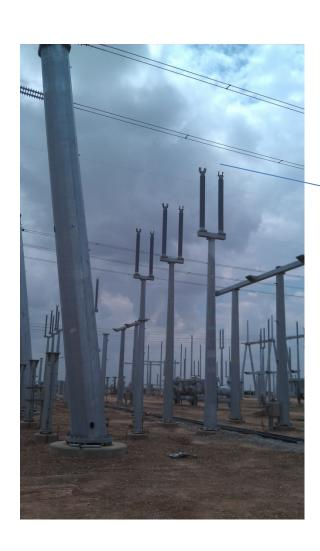
The very top of the insulators has a support that will eventually get a 6" aluminum pipe place in it. That pipe will carry the electricity that is dropped from the string bus by jumpers.
