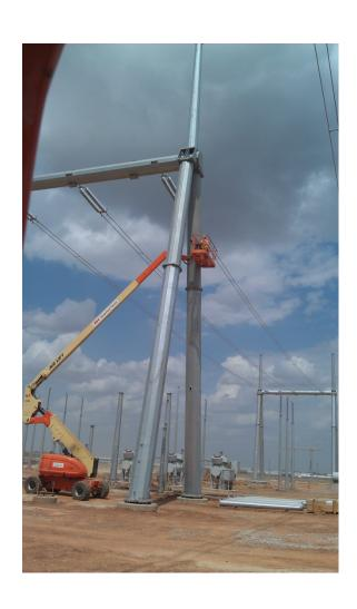
Foreman installing the mounting horns on the dead-ends for the station lights.
