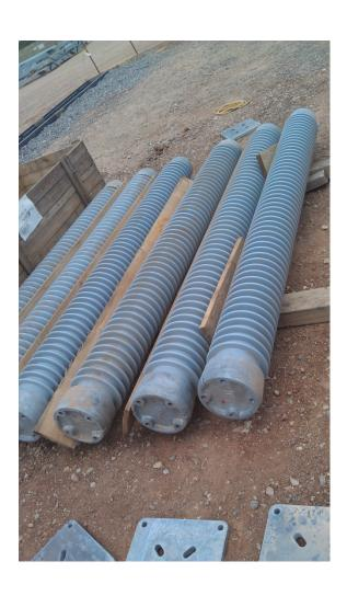
Insulators 6337: these particular ones will get the plates seen in the picture attached to the bottom. They will then be put on either a high or a low double.
