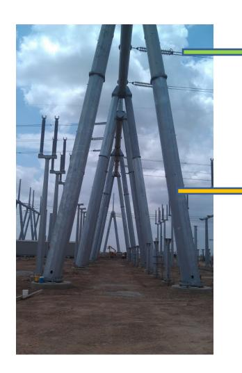
String bus: carries the electricity that comes into the station. The electricity will be brought to the aluminum pipe that runs on top of insulators attached to the steel. It is brought down using jumpers welded onto it. Hangs at 80ish feet off the ground.
