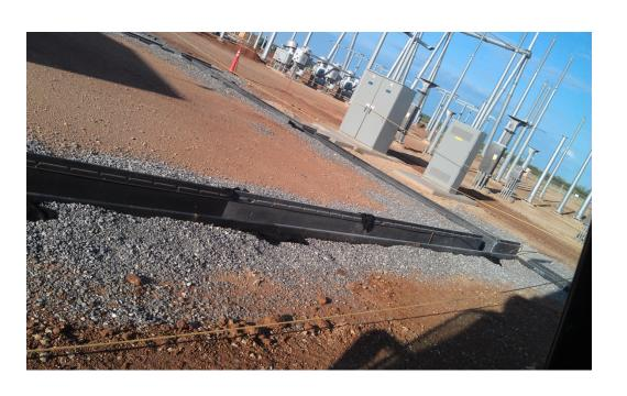
Cable trench: a cable tray will be covered eventually but this runs around the control building and also a north to south run on both sided of the site.
