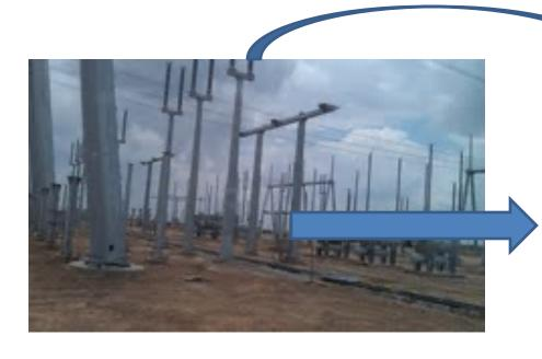
High Double bus support: single structure that has two insulators mounted on top.
