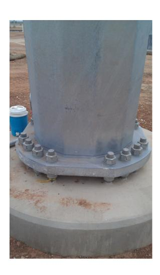
Pier for a dead-end structure. The pier is six foot in diameter and is 26 feet deep.
