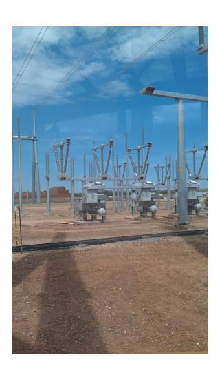
A completed v-type switch: the middle insulator is able to swivel and a motor operated switch is used to divert the direction the a b c phase electric current.
