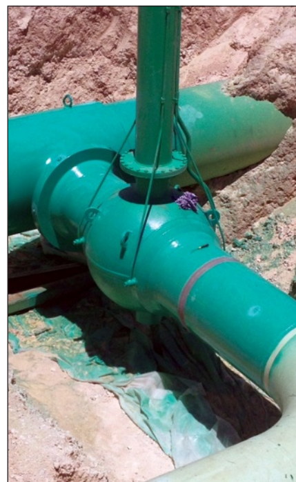
Fig. 5 — Completed hot tap ready for backfill.
