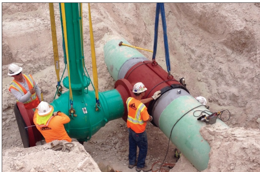
Fig. 1 — Hot tapping allows for a pipeline for be repaired or modified without interrupting service.
