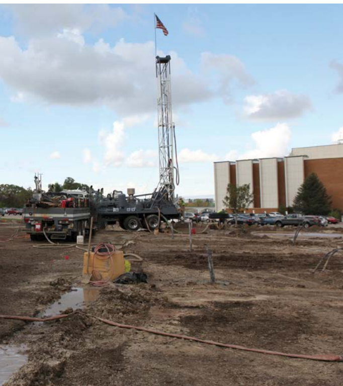
Crews work to bore deep-water wells below the parking lot on the north side of the stadium.
