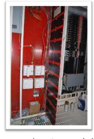
The new equipment uses much cleaner Cat-5 connections
