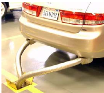
Exhaust Removal System
